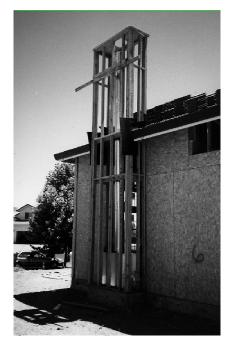
Figure 7-7 Factory-built flue and light-frame enclosure.
