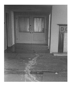
Figure 3-13 Example of damage caused in building on cut and fill site.
