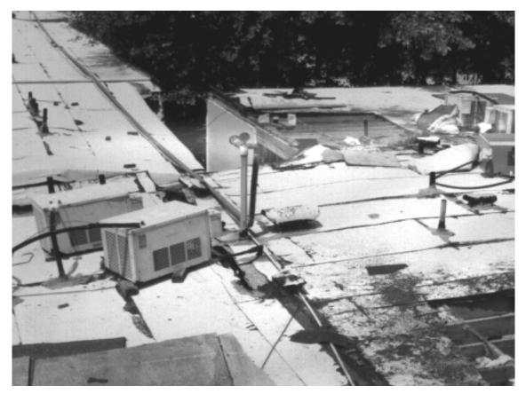
Figure 2-12 Roof-level damage to building with a T-shaped plan. The damage at the roof corner (right-hand side) is due to stress concentrations where the wings of the building connect.
