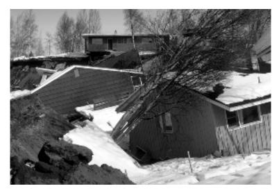
Figure 1-7 Houses damaged due to a landslide at the site. Photo Courtesy National Information Service for Earthquake Engineering, University of California, Berkeley
