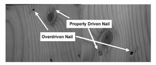
Figure 5-8 Properly and overdriven nails.
