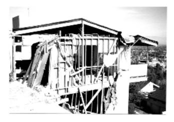
Figure 9-10 House located on a hillside site damaged during the Northridge, California, earthquake.
