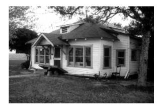
Figure 9-5a House with collapsed cripple walls. Photo Courtesy of National Information Service for Earthquake Engineering, University of California, Berkeley
