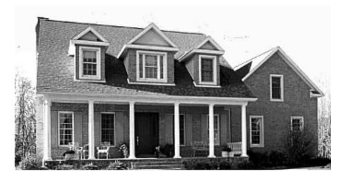
Figure 5-14 House constructed with masonry walls.
