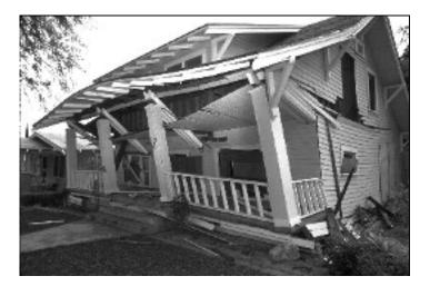
Figure 9-5b A house with severe damage due to cripple wall collapse. Photo Courtesy of FEMA.
