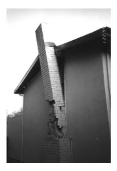
Figure 7-2 Chimney damage in Northridge earthquake.
