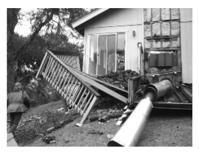
Figure 7-8 Collapsed factory-built chimney, light-frame enclosure, and deck after the San Simeon earthquake. Photo courtesy of Josh Marrow, Simpson Gumpertz and Heger Inc.
