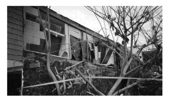
Figure 5-12 Stone veneer damaged during the earthquake in Northridge, California.
